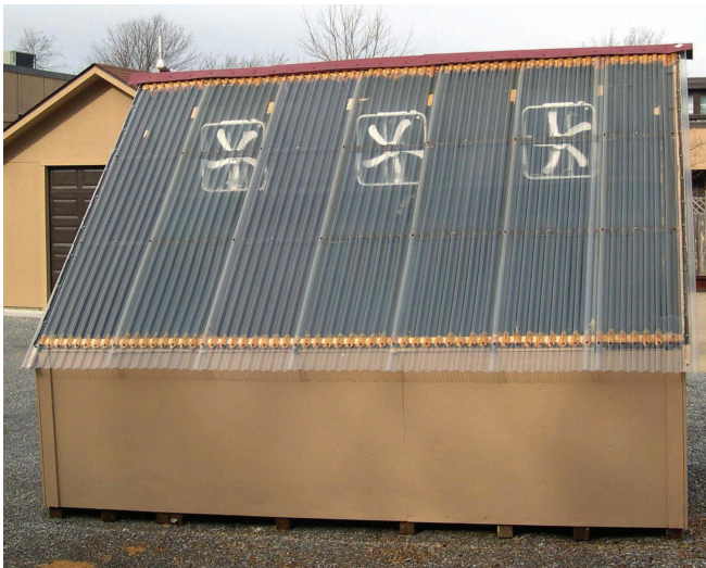
Figure 5—Front view of kiln showing fan placement.
