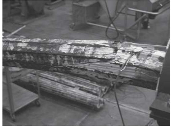
FIG. 5. The failure of a uniform diameter hollow wood laminated composite pole without inserted node-like plywood webs when subjected to a cantilevered bending.
