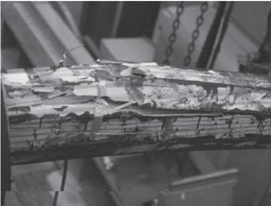
FIG. 4. The failure of a uniform diameter hollow wood laminated composite pole with inserted node-like plywood webs when subjected to a cantilevered bending.
