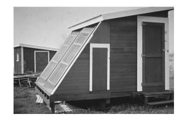
*Figure 11.* East side of solar lumber dryer showing principal loading and unloading door and the small access to collector area. (Photo courtesy of USDA Forest Products Laboratory).
