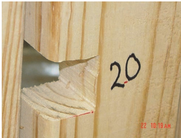
Figure 4. Termites were active in the machined areas of the samples. Note the termite activity in the notch of the Sample 20 (untreated control).
