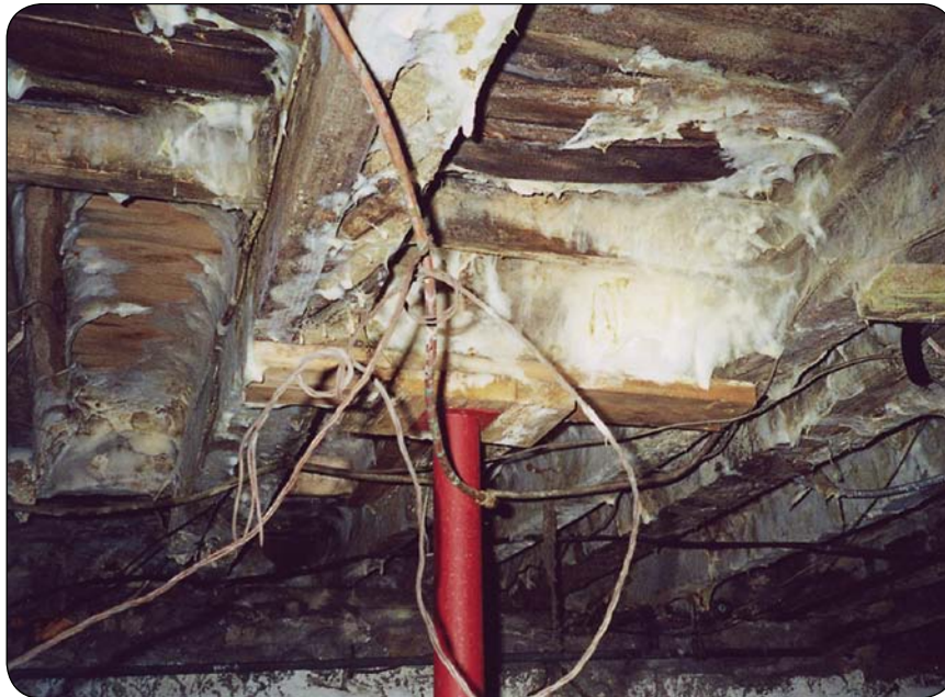
Dry rot starts when an infected piece of wood forms a bridge between soil and other wood in a house. (Photo by Carol Clausen, FPL.)
