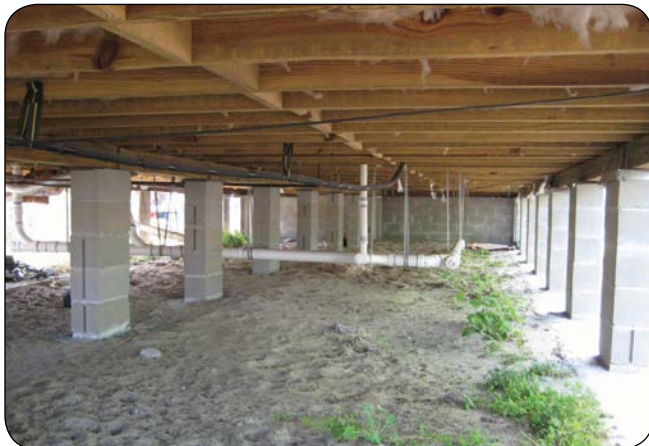
Open pier-and-beam crawl space generally does not need a ground cover. (Photo by Samuel Glass, FPL.)
