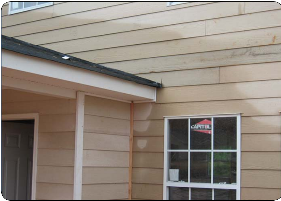
Without kick-out flashing and proper gutter placement, water flowing off the roof runs down the siding. (Photo provided by Steve Easley, Steve Easley & Associates, Inc.)
