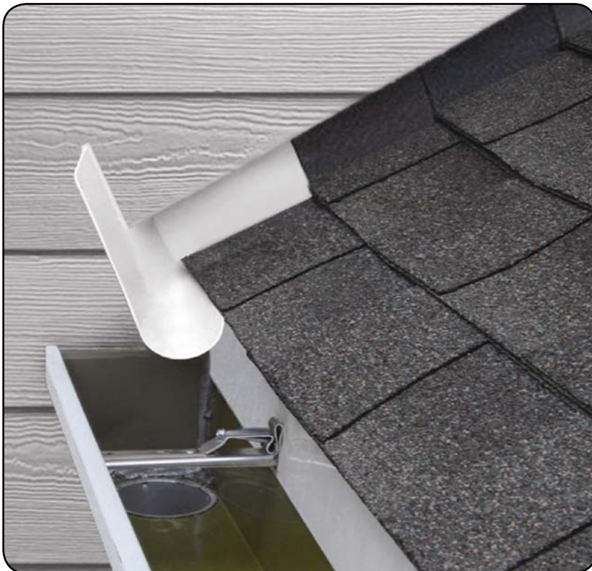
Properly installed kick-out flashing. (Photo provided by Scott Butler, DryFlekt Products, Inc.)
