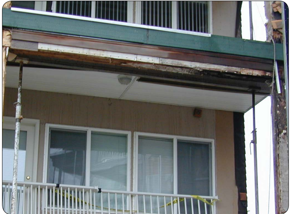
Joints that trap water and dry slowly are prone to decay. (Photo by Lonnie Houghton.)
