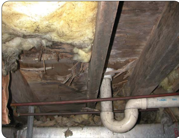
Decayed subfloor and floor joists. (Photo provided by Advanced Energy, Raleigh, N.C.)
