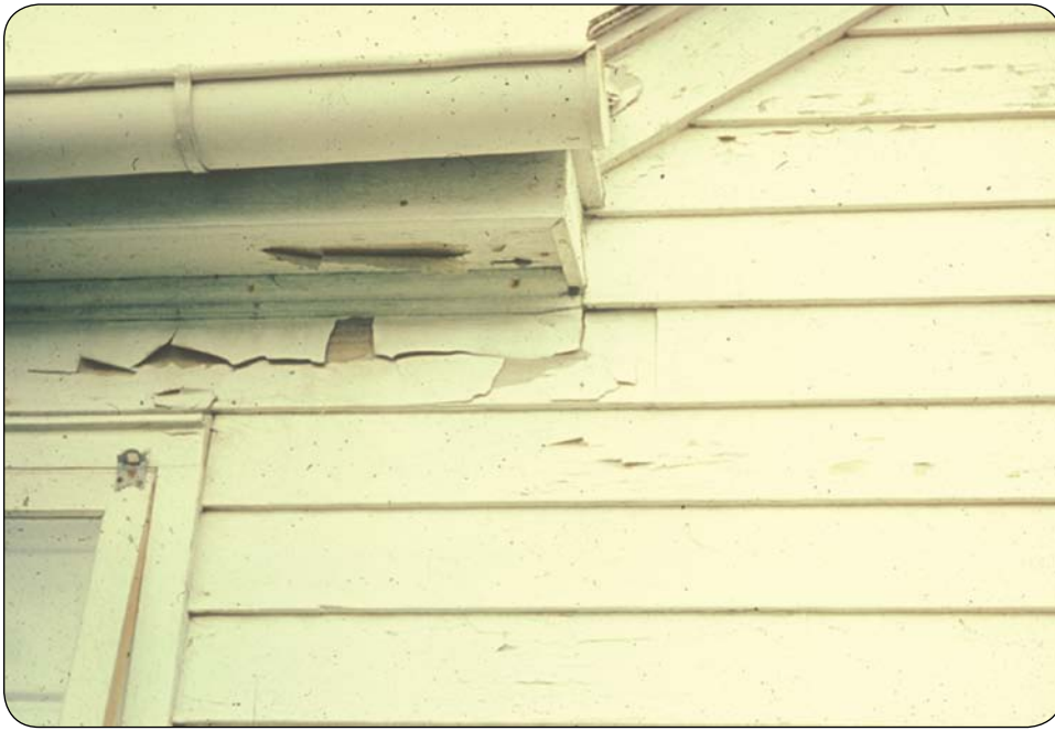
Water running around roof edges and onto wood below can get trapped in joints and is absorbed rapidly at cut ends of wood trim and beams. Paint failure and decay begins at these points.
