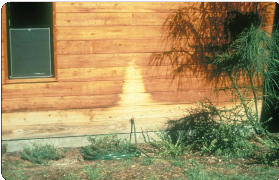
A high-decay hazard can be artificially created when wood siding is repeatedly wetted by a lawn sprinkler, faucet, or vegetation that is planted too close.
