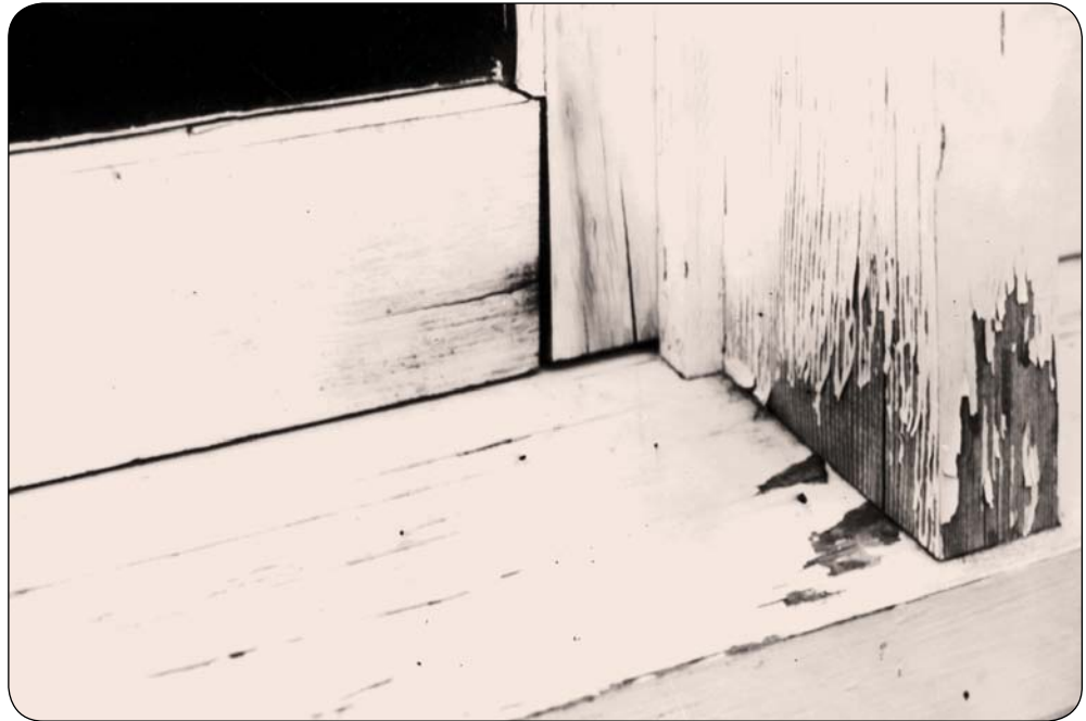
Wood resting directly on a sill makes it prone to decay.
