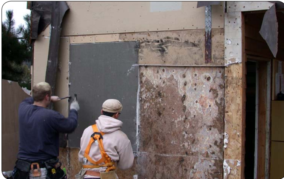
Improper installation of flashing, sheathing, and trim can lead to absorption of water by building materials and hidden decay inside the wall cavity of the structure. (Photo by Carol Clausen, FPL.)
