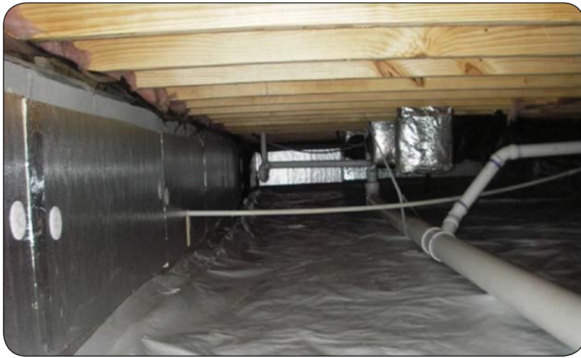
Polyethylene ground cover professionally installed. (Photo provided by Advanced Energy, Raleigh, N.C.)
