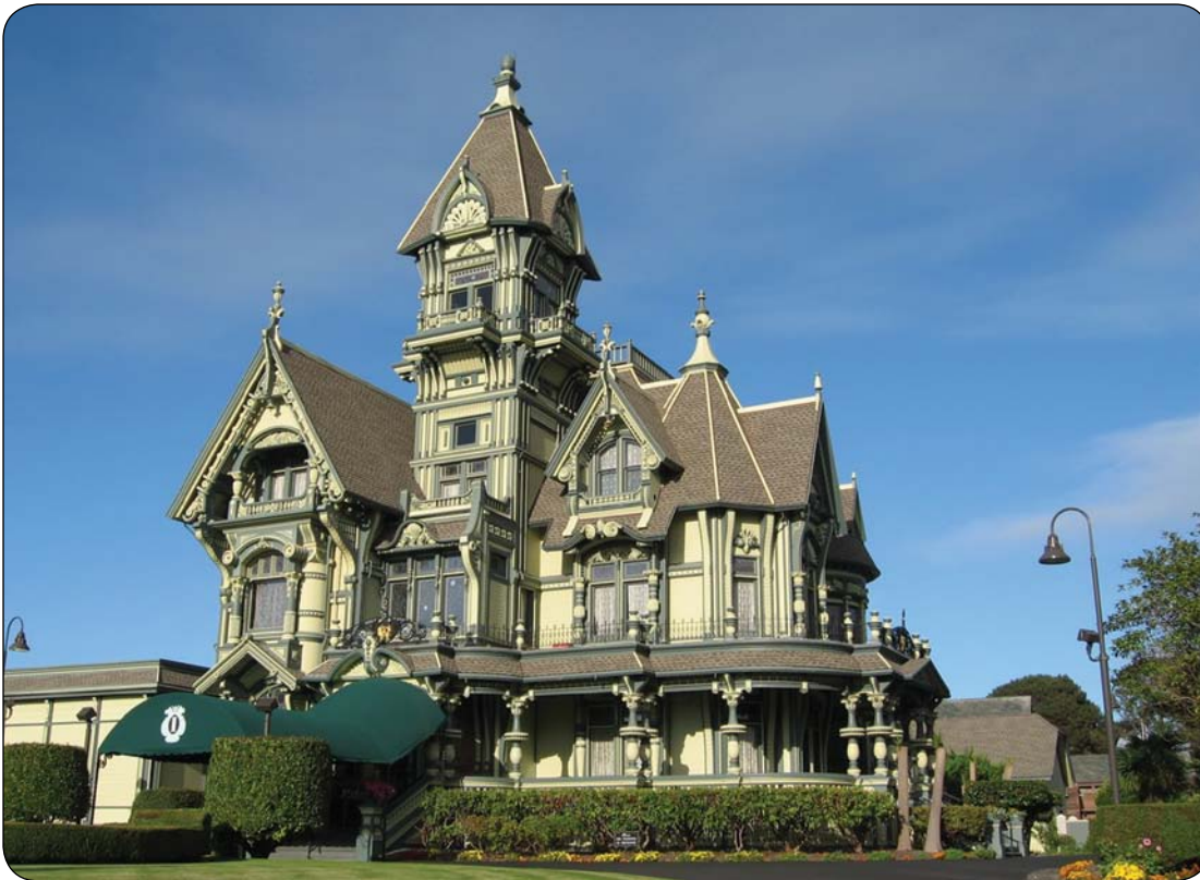
The Carson Mansion in Eureka, California, built in 1884, is just one example of magnificent west coast Victorian structures constructed during the late 19th century that are still in service. (Photo by Carol Clausen, FPL.)
