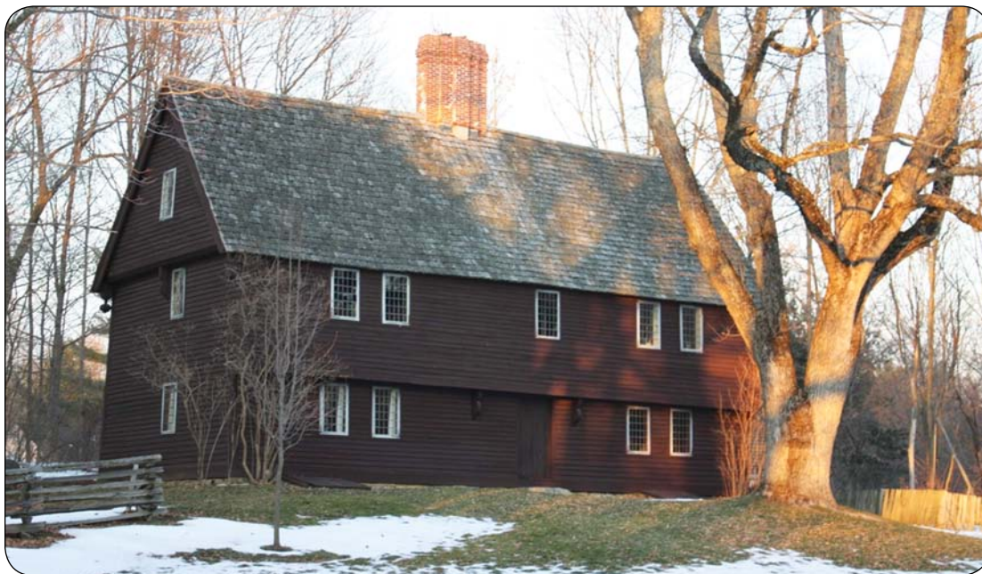
The Parson Capen House was built in 1683 in Topsfield, Massachusetts. The building design and construction detail that do not allow water to collect are fundamental features that have contributed to over three centuries of service by this house. (Photo provided by the National Park Service.)
