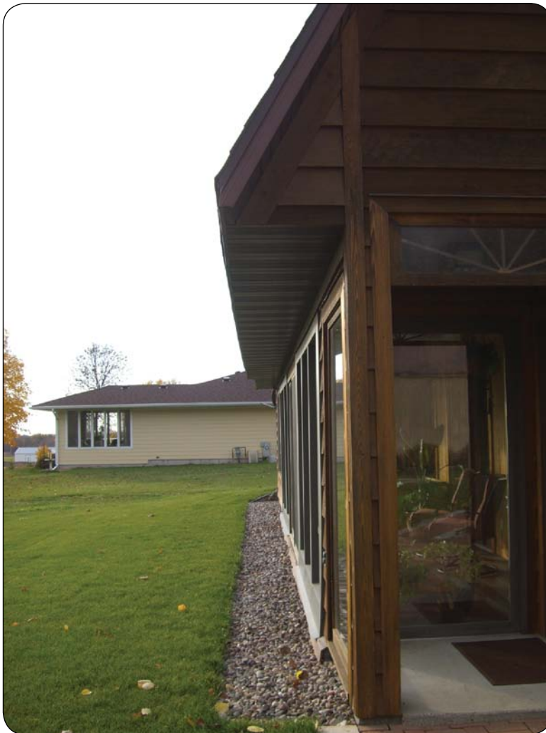
A wide roof overhang directs water runoff from the roof away from the exterior walls. The splash zone is also moved farther away from the building. (Photo by Carol Clausen, FPL.)
