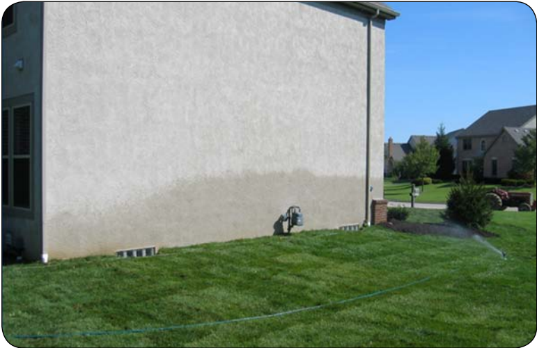
Soil graded high against the exterior brick veneer (above) will contribute to decay problems in untreated wood members below the grade line. Similar problems will occur with soil graded high against stucco and siding. The finish grade on the yard (below) is above the level of wood framing inside the wall. To make matters worse, the lawn sprinkling system is providing constant wetting of the stucco siding on this home. (Photo provided by Steve Easley, Steve Easley & Associates, Inc.)
