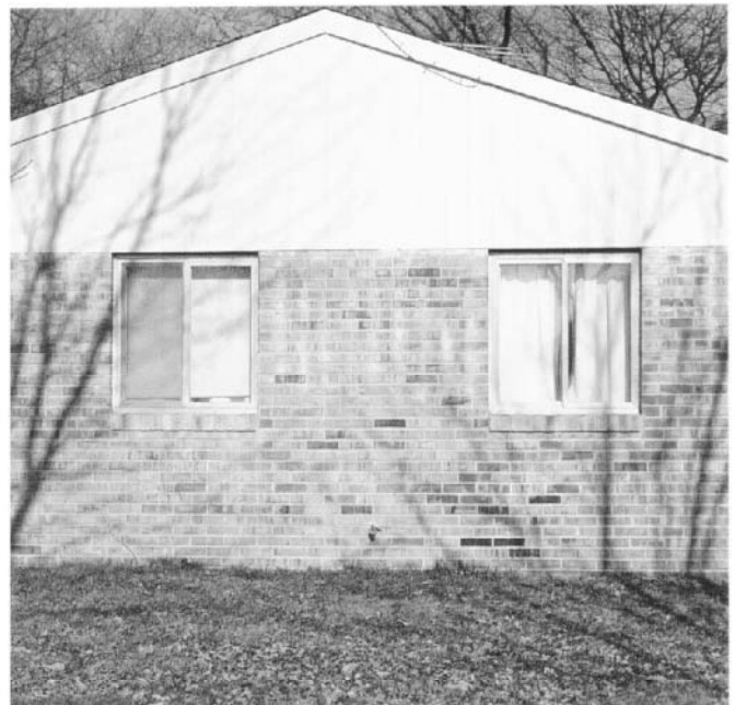
Figure 38—Chalking of paint. Some paints or stains chalk badly. Chalking can discolor a lower surface as the resin and pigment particles wash down.
