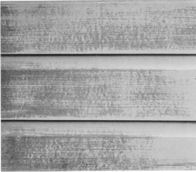
Figure 32—Mildew on paint is most common in warm, humid climates. It also occurs in shaded or protected areas.
