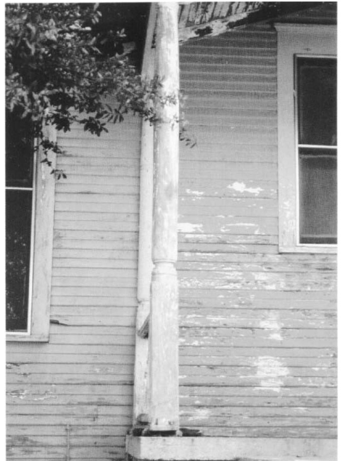
Figure 36---Paint can peel from wood when excessive moisture moves through the house wall. Some cross-grain cracking is also evident on this older house. (Photo courtesy of Southern Forest Products Association.)
