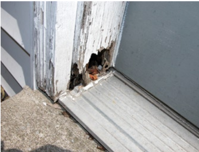
Figure 13B—Extensive jamb decay in a contemporary exterior entry door. The decay was in all likelihood exacerbated by the short length of fillet joint that blocked drainage at the outside lower edge of the jamb.
