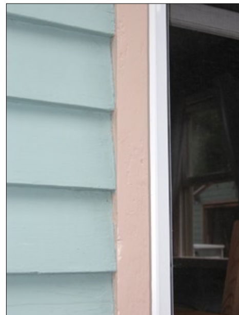
Figure 1B—Painted redcedar lap siding butting tightly against a window casing without caulk. Photograph taken summer 2005 on a single-story home built in 1940.
