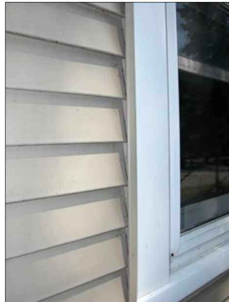
Figure 4A—Vinyl siding terminating in a J-channel receptor along window jamb trim.
